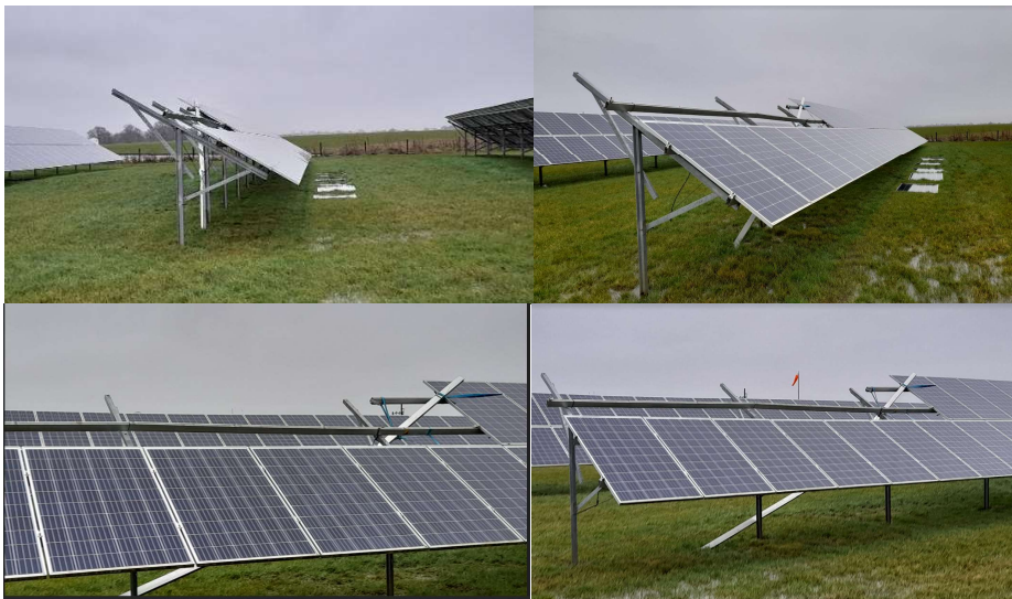
Wind Damaged Area at NBJ Prior to Repair
