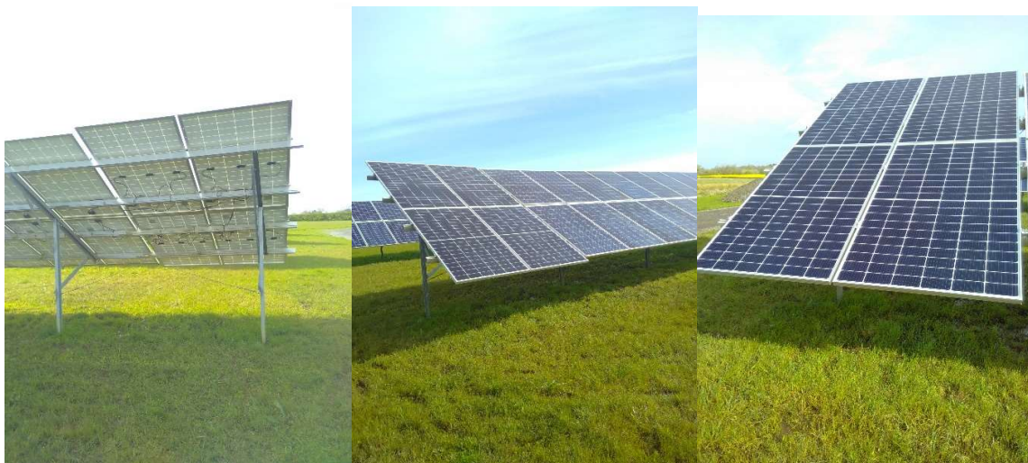
NBJ Post Repair To Wind Damaged Area – Note 4 slightly larger replacement panels
